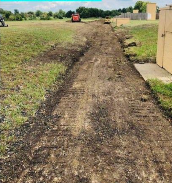
Grading Trap House access to allow water to flow into creek without flooding the houses. 08/18/22
